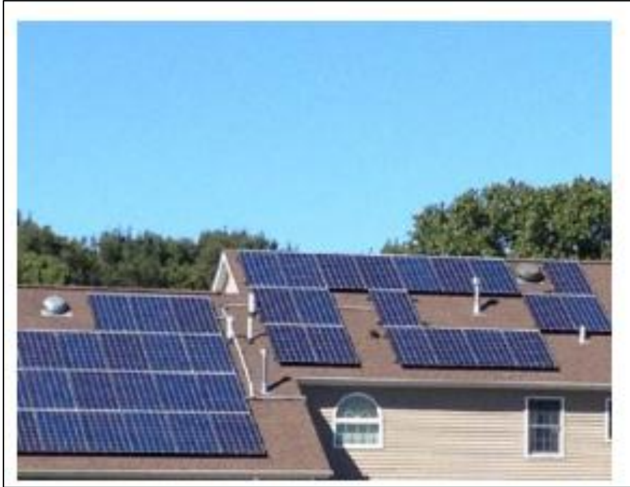
A disjointed arrangement of panels.
