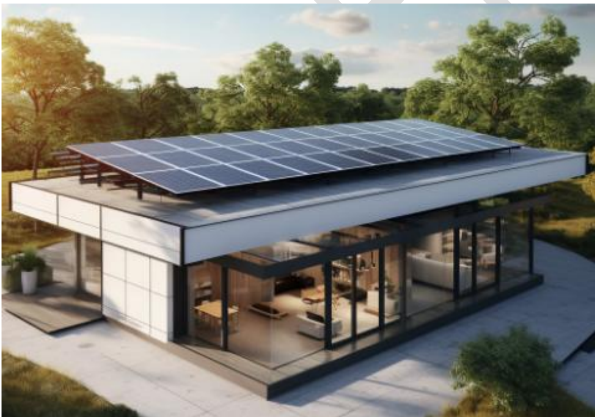
Panels on a flat roof without a parapet, mounted in an organized pattern, parallel with the edges of the roof.
